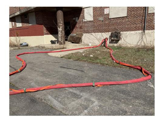
Continue down the hose connecting each tether as you go. The 3 red tethers will end up at the standpipe end of the hose.
