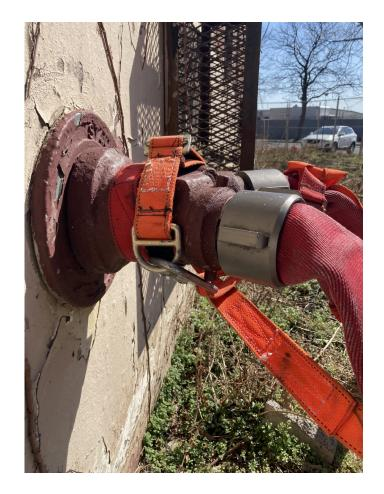
The end of the hose with the 3 red tethers will connect to the standpipe tether.
